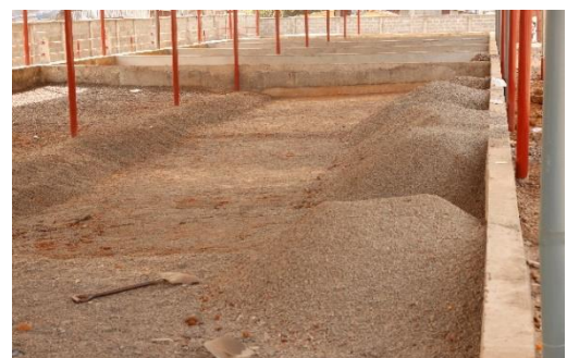
Remodelling of drying beds to install Geobags
