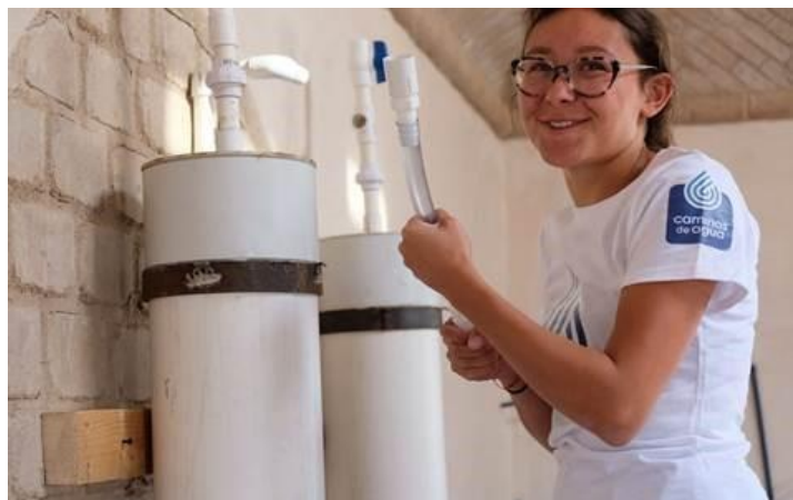
Johanna involved in the design and construction of a groundwater treatment system
